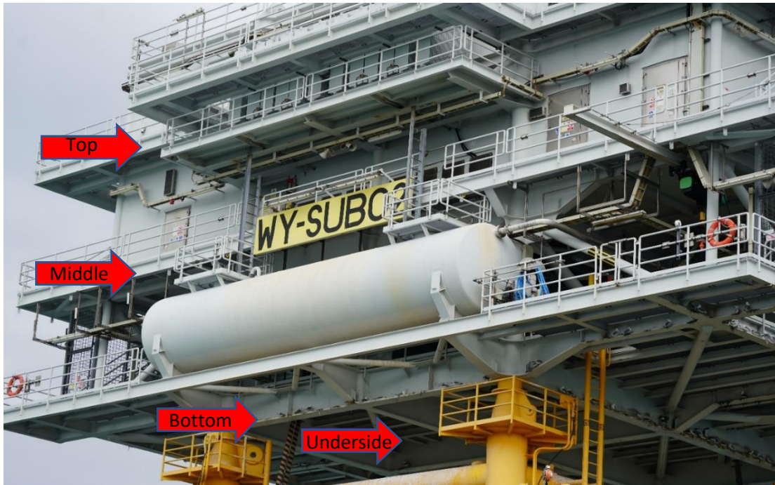
Figure 4: South side of the substation divided into layers based on height.
