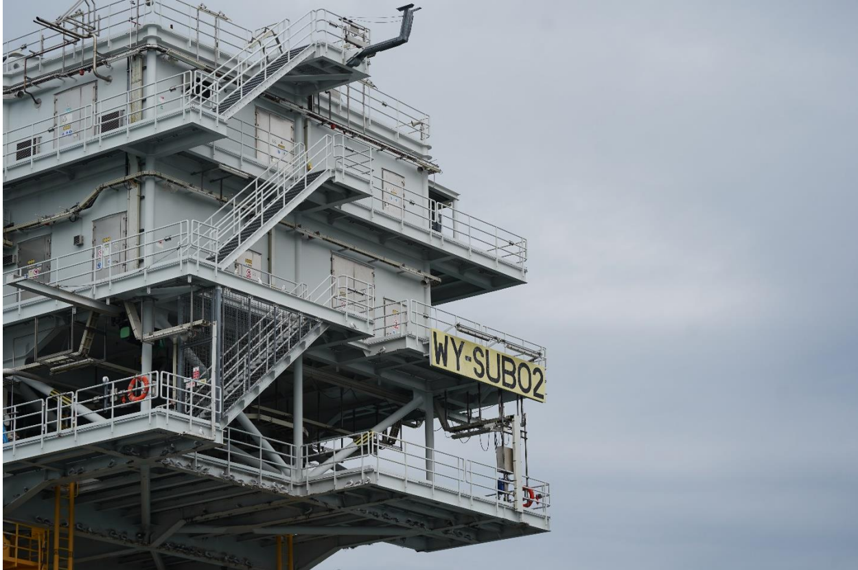
Figure 3: Whole aspect photo of the southeast corner of the substation (taken 18 th August 2023).
